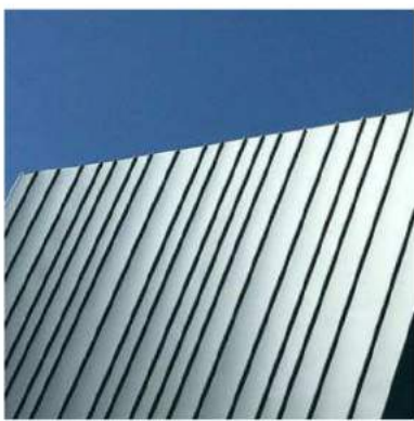
CHARCOAL RANDOM SEAM METAL CLADDING CL-03
