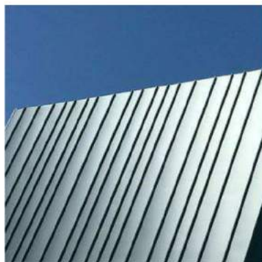
CHARCOAL RANDOM SEAM METAL CLADDING CL-03
