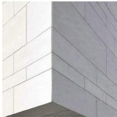
OFF WHITE EXPRESSED JOINTED PANEL CLADDING FC-02
