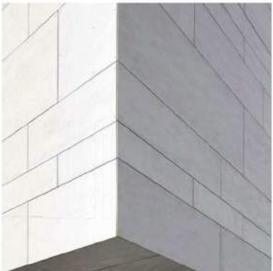
OFF WHITE EXPRESSED JOINTED PANEL CLADDING FC-02
